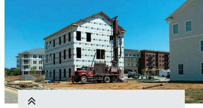
Geothermal heat pump drilling at a new housing development in Norton Commons, North Village, Kentucky. *Photo by Norton Commons*
