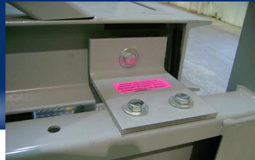
Seismic Restraint and Shipping Tie Down
